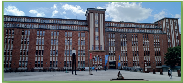
Exterior view of the CCH building
